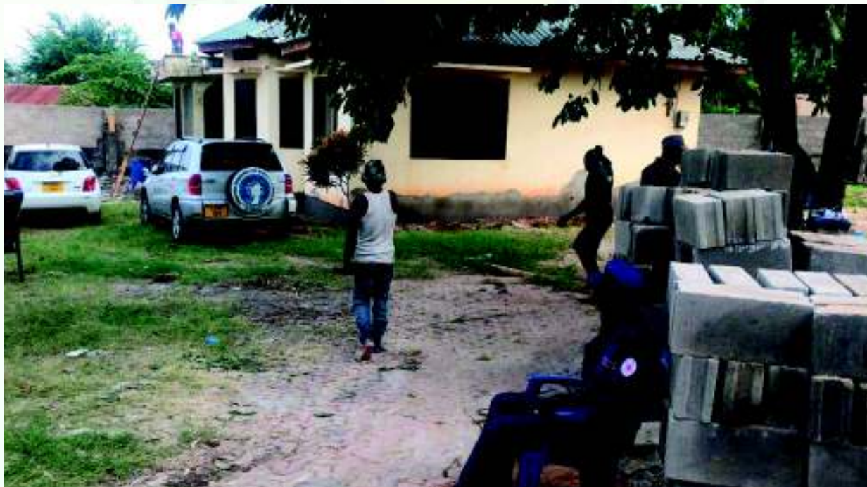
Renovation continues at the newly acquired in January 2021
